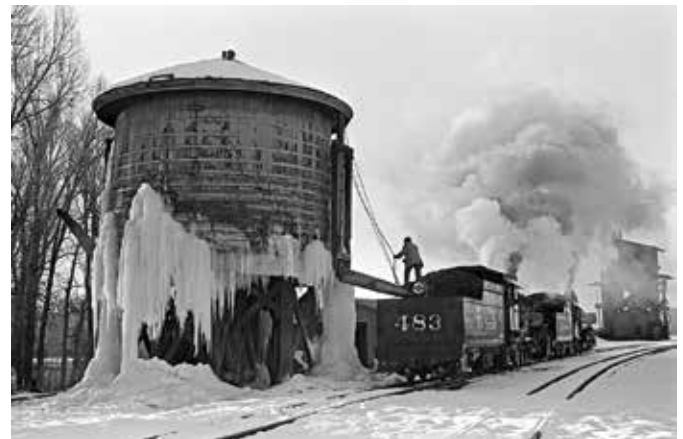
D&RGW #473 getting ready to continue from Chama to Durango with the last westbound freight of the D&RGW narrow gauge line, Chama, NM. Photo by Ernie Robart December 6, 1968 FCTS ERNG19681206
