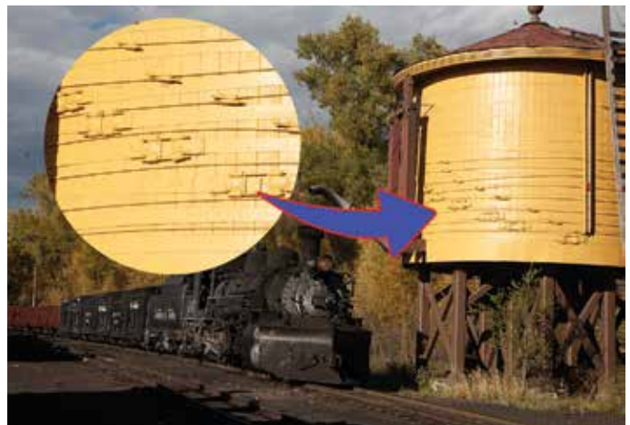
On the restored tank, you can clearly see the original banding and brackets on the bottom portion of the tank.
