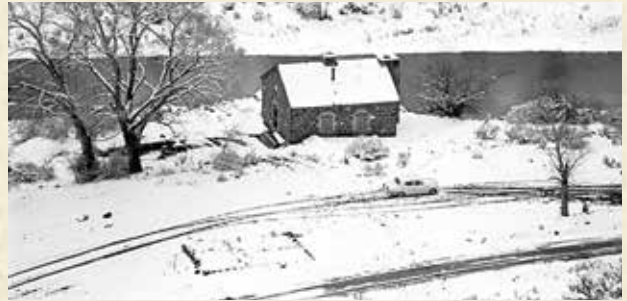
View of the Pump House below the tank, April 1968. Note the old foundation of the "Pumper's Dwelling." Photo by Ernie Robart FCTS ERNG19680423-1676
