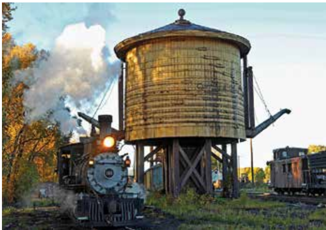
Chama Tank, upright again. 2016. Photo by Don Atkinson
